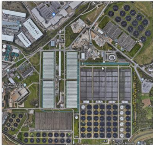
London, Beckton, Thames Water, 3,5 Mio EW, ASP3 8 Kanal N-RTC, SRT-RTC Installation
