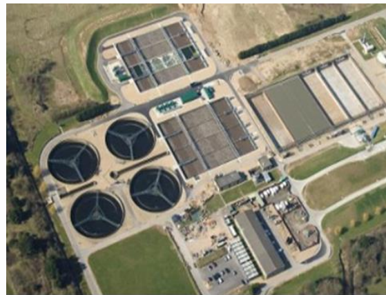
Southampton, Southern Water, 250.000EW N-RTC, DN-RTC, SRT-RTC Installation
